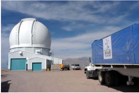
The final stages of construction of SOAR: the primary mirror in its supporting cell (with 120 activate supports). The arrival of the first (of several) trucks carrying the optics and support structures at the SOAR dome.
